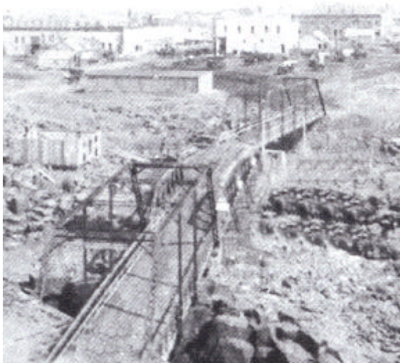
Eagle Rock's (Idaho Falls) 1 st Steel Bridge
